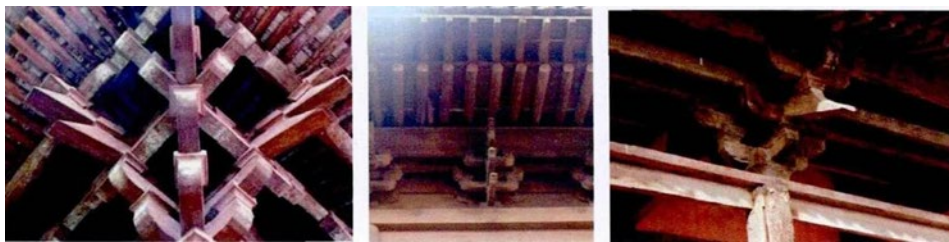
Figure 3 From left to right, corner bucket arches, inter-column bucket arches, and column head bucket arches
